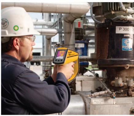
By using thermal imaging, Alltech determined that insufficient airflow and cooling was causing this pump seal to fail, saving a \$100,000 project from ongoing seal failure.
